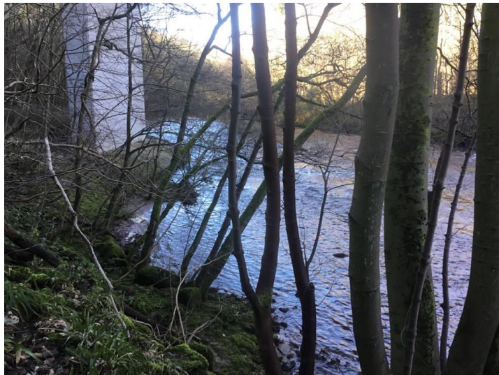
Photograph 1: South pier looking upstream to river training works and position of the new pier
