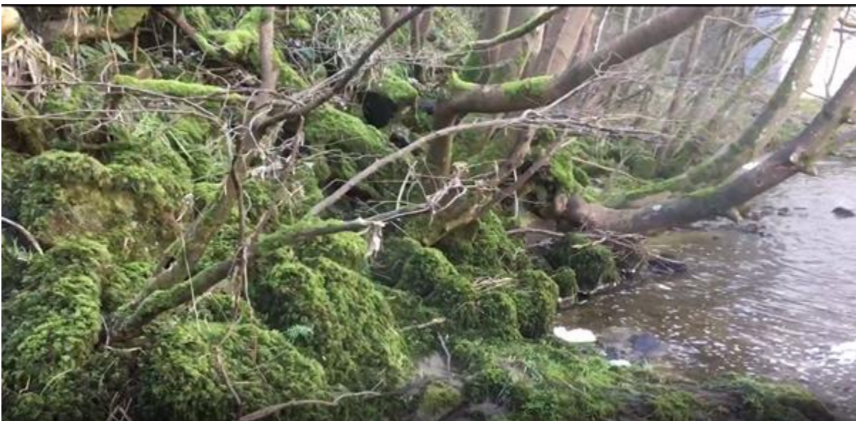
Image 3. Boulder sized material with trees along south bank (view of looking upstream along south bank to existing pier)
